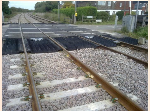
Rail track crossing reinstated with UltraCrete products
